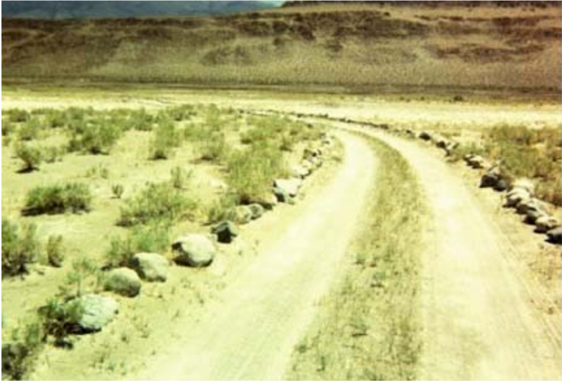
EXHIBIT 4-6 ROCK BARRIER ON FISH SLOUGH ROAD (photo from June 2, 2004)
